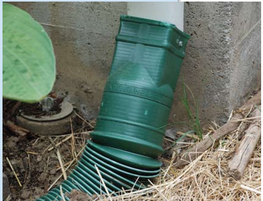
Figure 14. Downspout connected to downspout extension that directs flow away from a building's foundation. Note sheet-metal screws.
